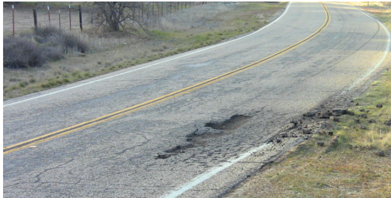
Figure MP 4.7-2 Road wear and tear Field Observation of solar traffic to the Carizzo
